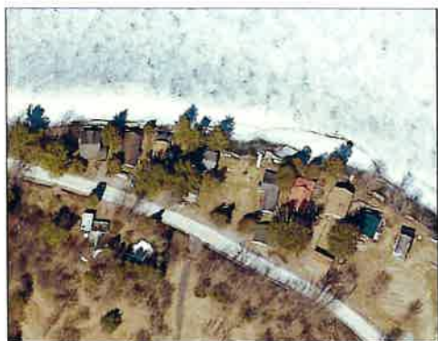
Dense development poses along the lakeshore poses planning challenges
