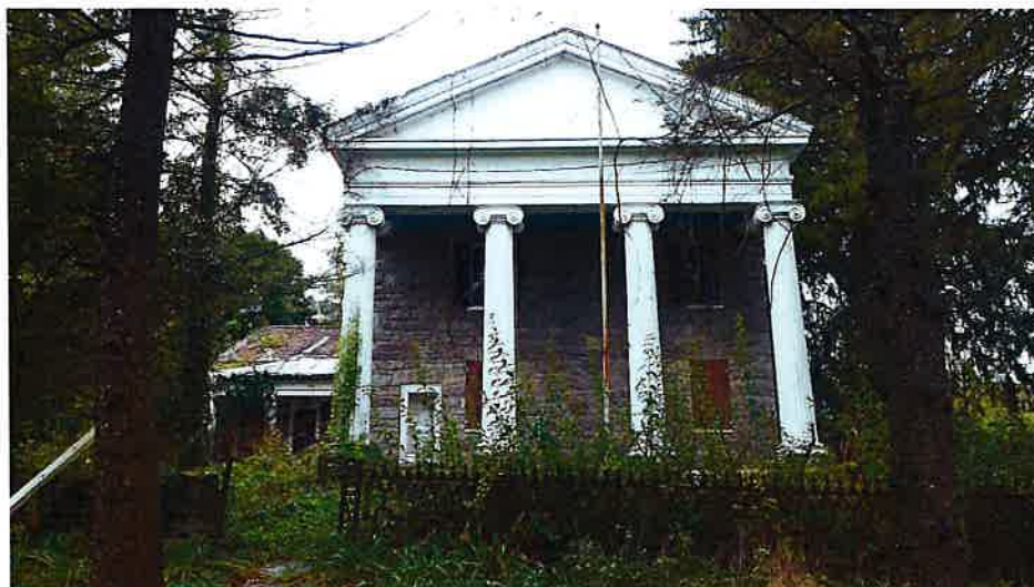
Clockwise from Top Left: The brick office building, the fire house, and the original stone Mott Morse House.
